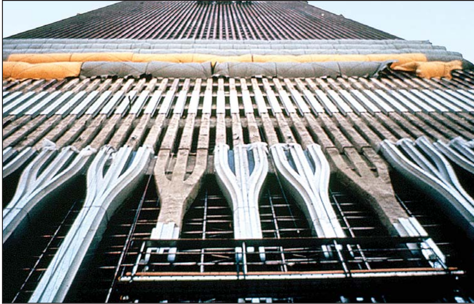
Figure 2-4 Base of exterior wall frame.
