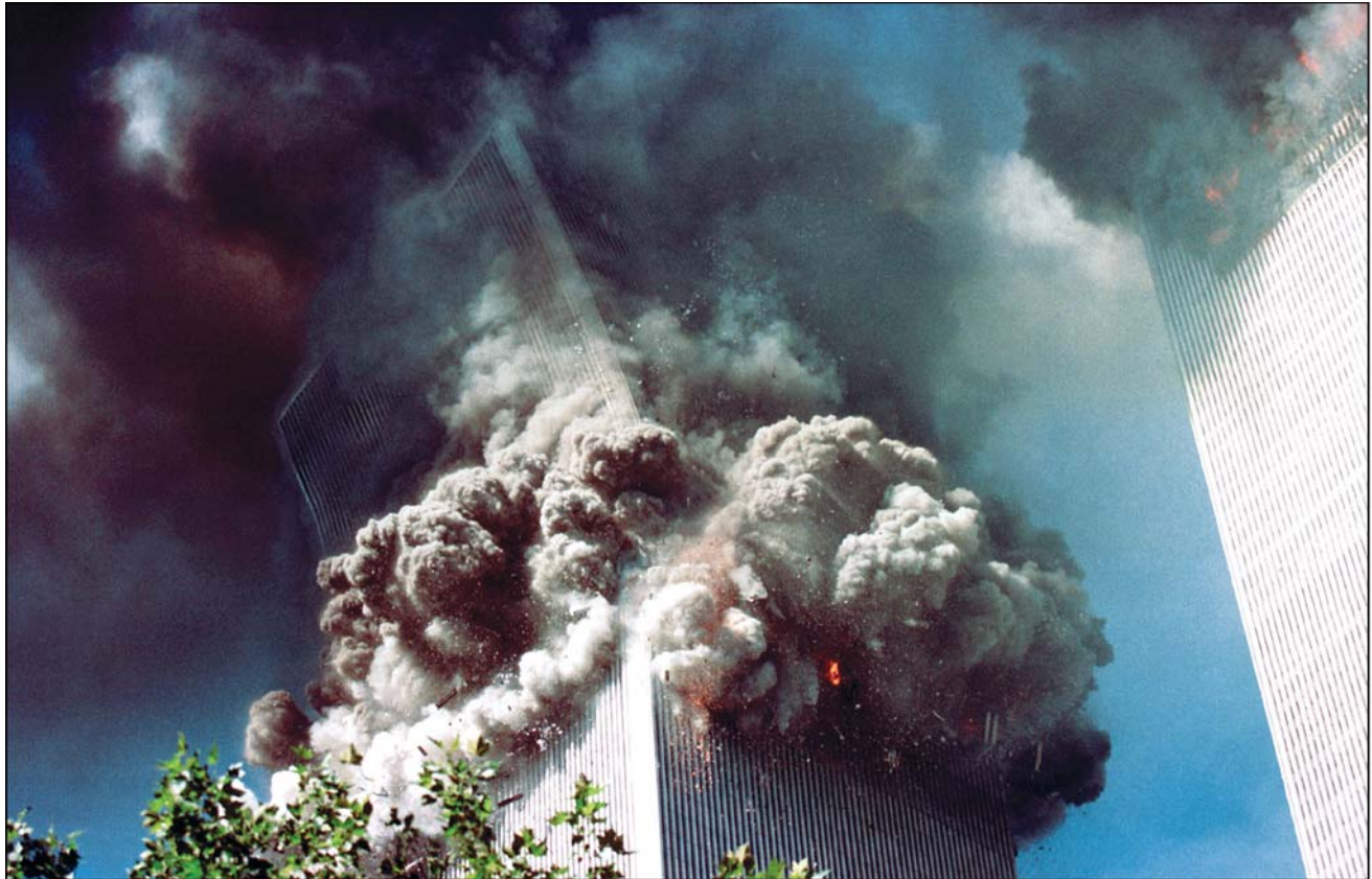
Figure 2-32 The top portion of WTC 2 falls to the east, then south, as viewed from the northeast.
